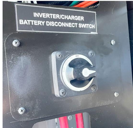
Inverter/Charger disconnect switch (located in the exterior compartment).
